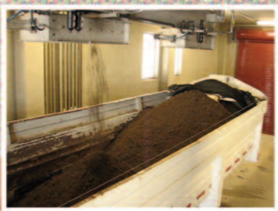
Water is removed from biosolids and the resulting “dirt” is trucked to a landfill
