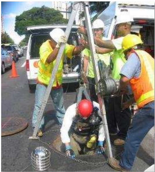
Photo 2-1. Confined Space Entry
