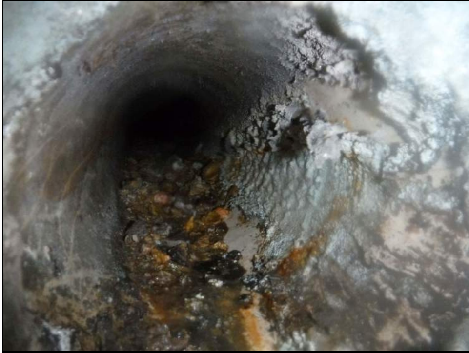
Northeast Influent Pipe
