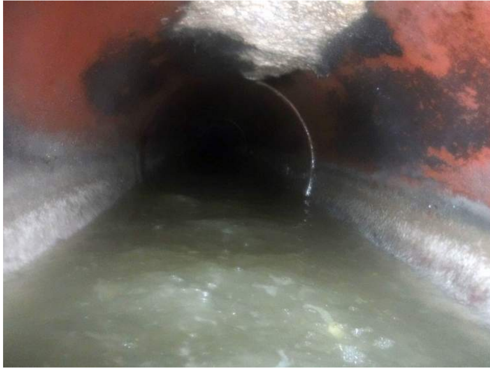
Northeast Effluent Pipe
