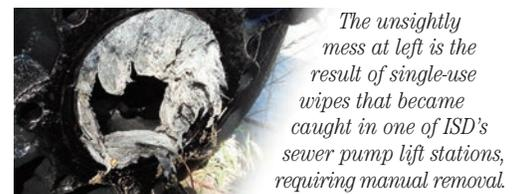
The unsightly mess at left is the result of single-use wipes that became caught in one of ISD’s sewer pump lift stations, requiring manual removal.
