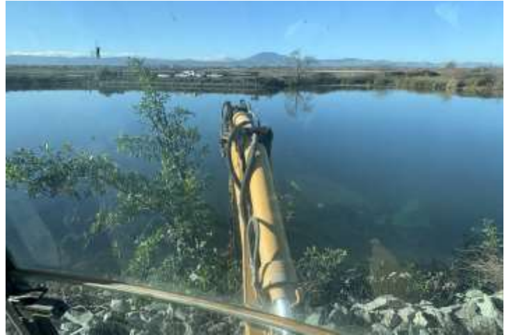
Removal of saplings from waterside
