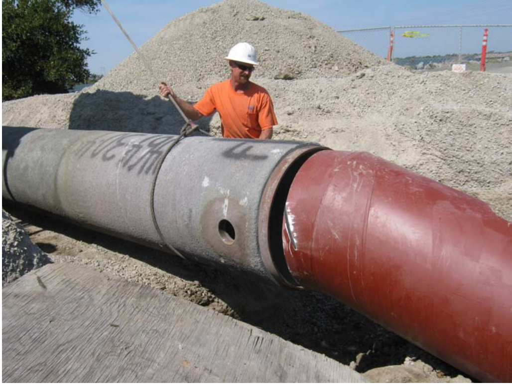
Final Connection at Jersey Island
