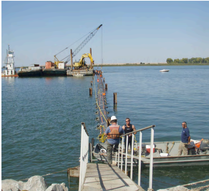
Outfall Pipe In Position Ready to be Sunk Into Place
