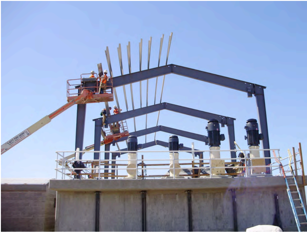
Structural Steel Installation at UV Structure Effluent Pumps Installed
