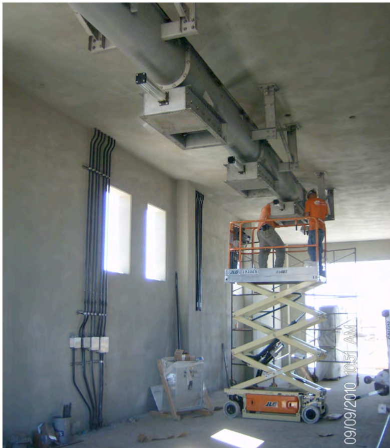
Overhead Screw Conveyor Installation at the Solids Handling Building
