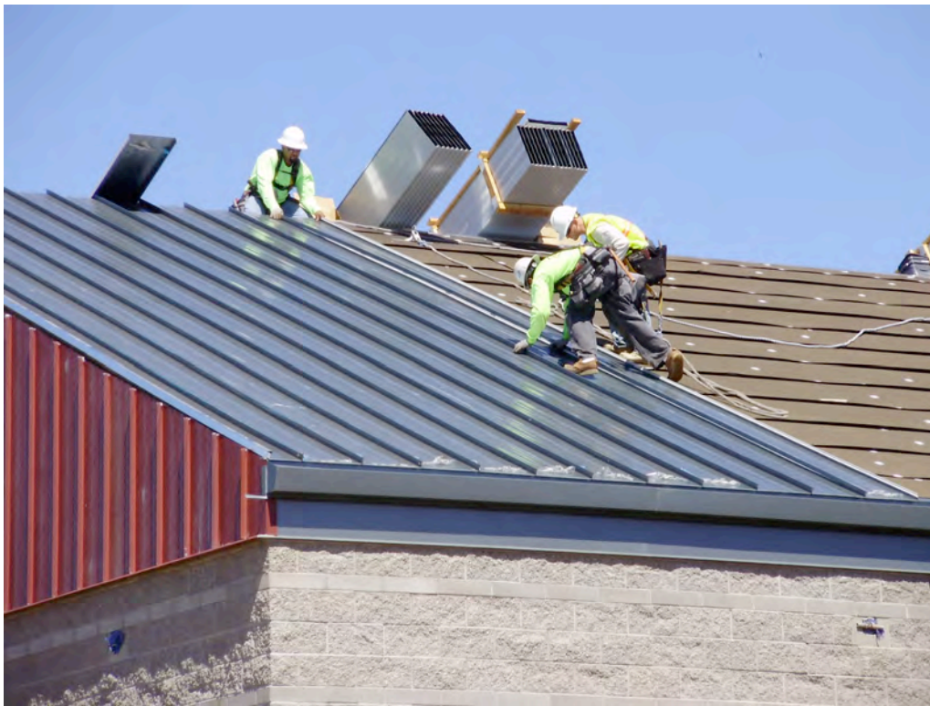
Chem/Blower Building Roofing Installation
