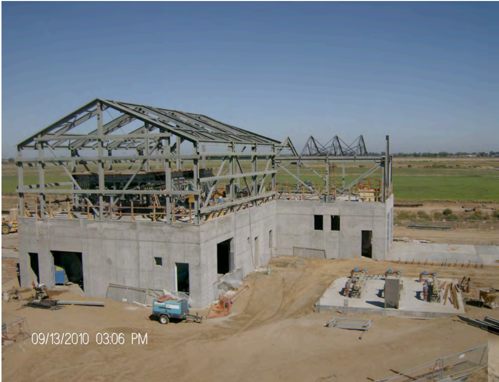
Solids Handling Building Metal Building Installation
