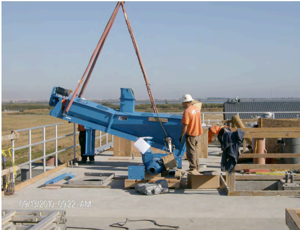
Grit Classifier Lowered Into Place on the Headworks Deck
