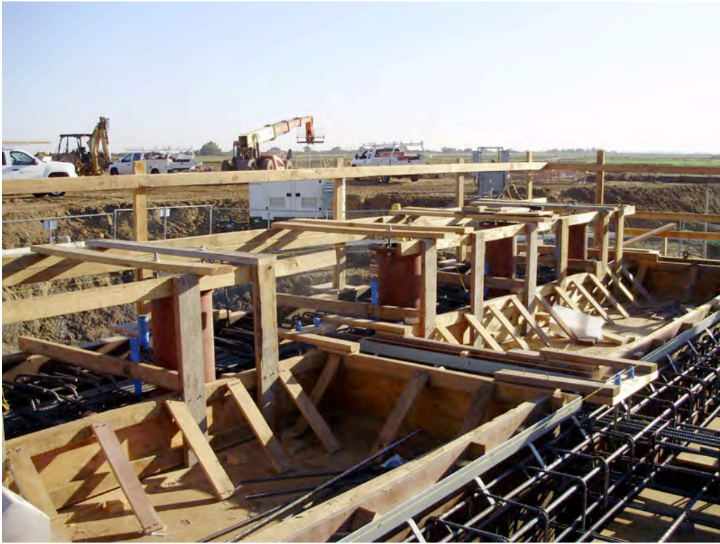
Rebar Installation at the Influent Pump Station Deck
