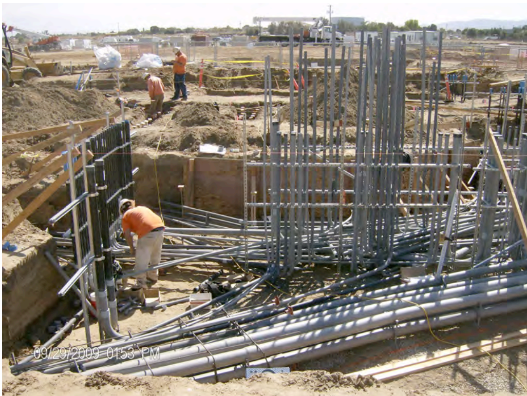
Conduit Installation at the Solids Handling Building
