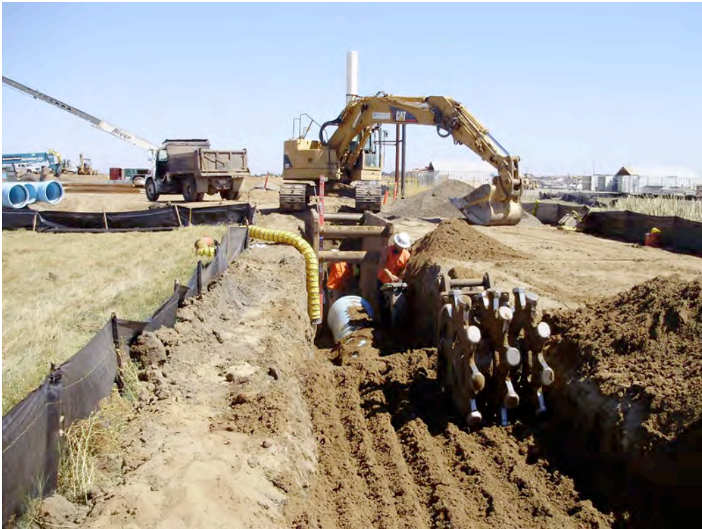
Backfilling 30" Overflow Pipeline
