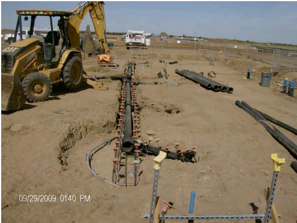
Below Slab Pipe Installation at the Solids Handling Building
