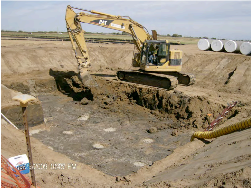
Excavation of the Effluent Pump Station
