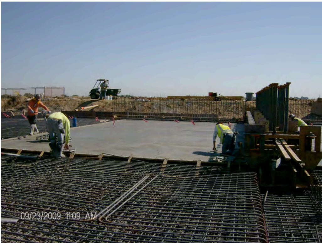
Concrete Finishing at the AA Basing Slab
