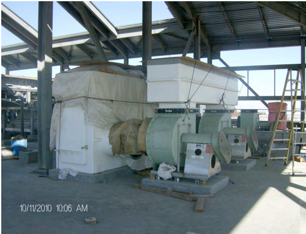
Solids Handling Building Odor Control Fan Installation
