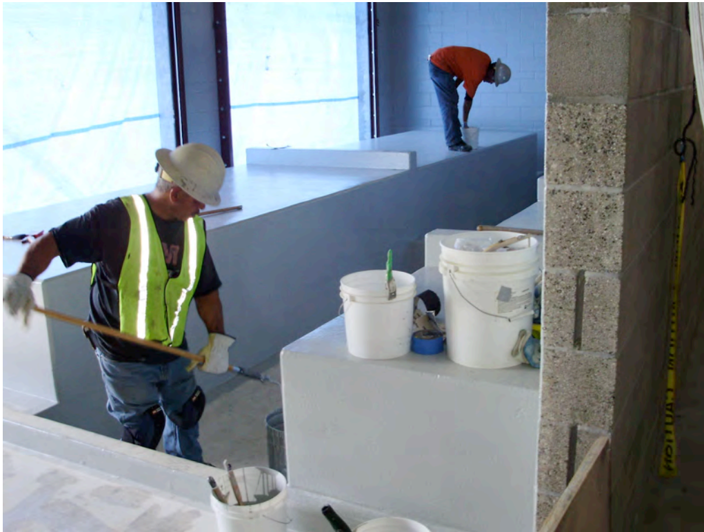
Coating the Chemical Area at the Chem/Blower Building
