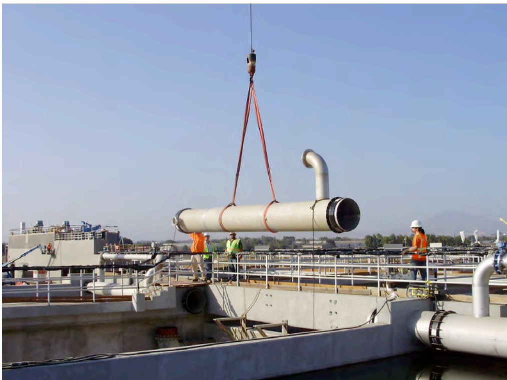
30" AA Basin Installation
