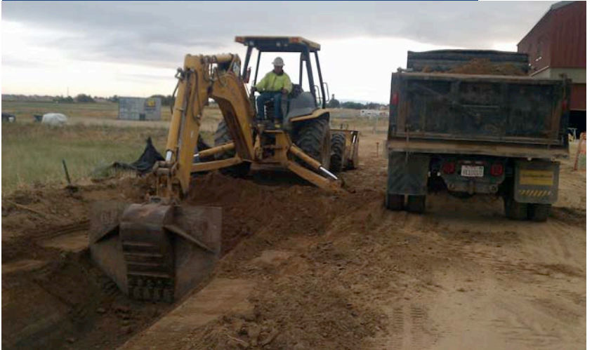
Installation of Storm Drainage Facilities
