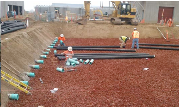
Installation of the Biofilters
