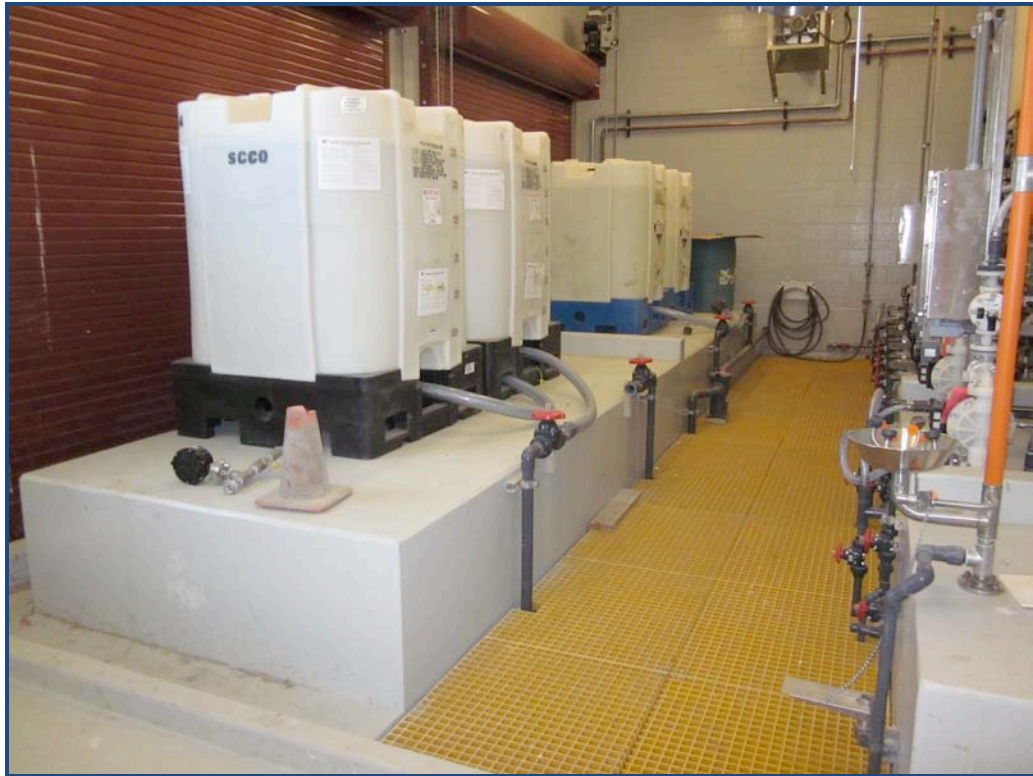
Chemical Totes Installed, Pumps Tested
