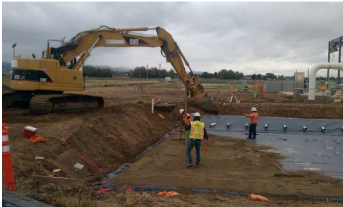
Installation of the Biofilters
