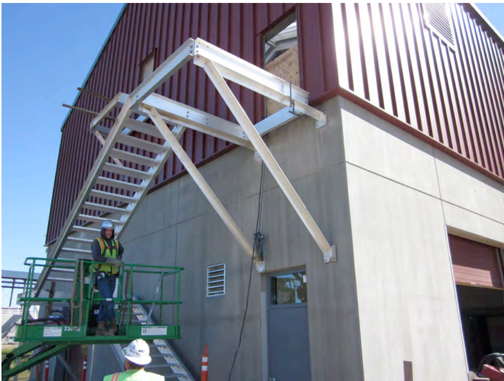
Exterior Stair and Landing Installation at Solids Handling Building
