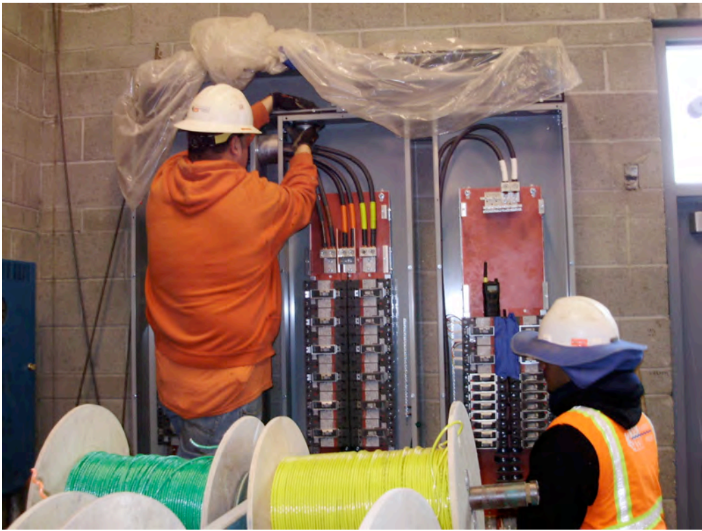
Wire Installation and Termination at Chemical/Blower Building
