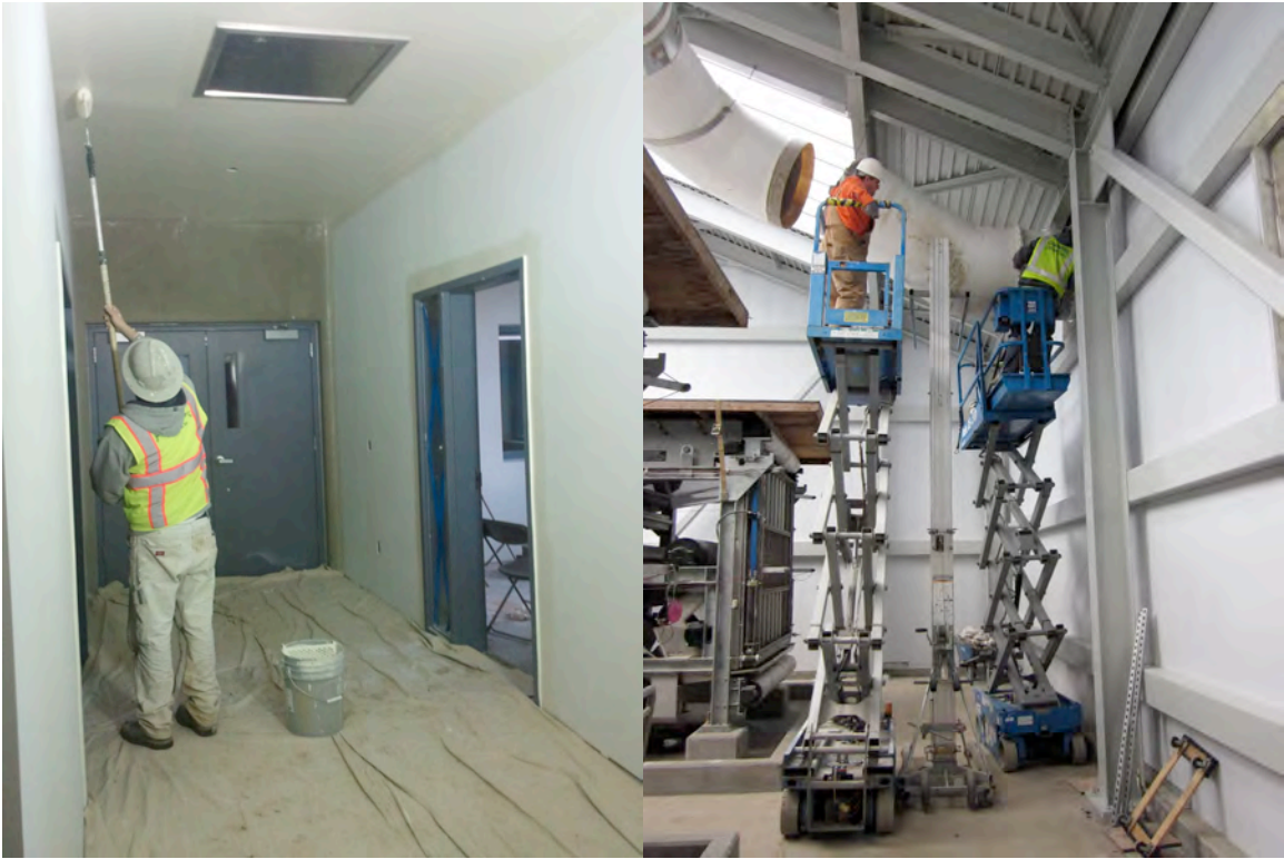
Painting and Duct Installation at Solids Handling Building
