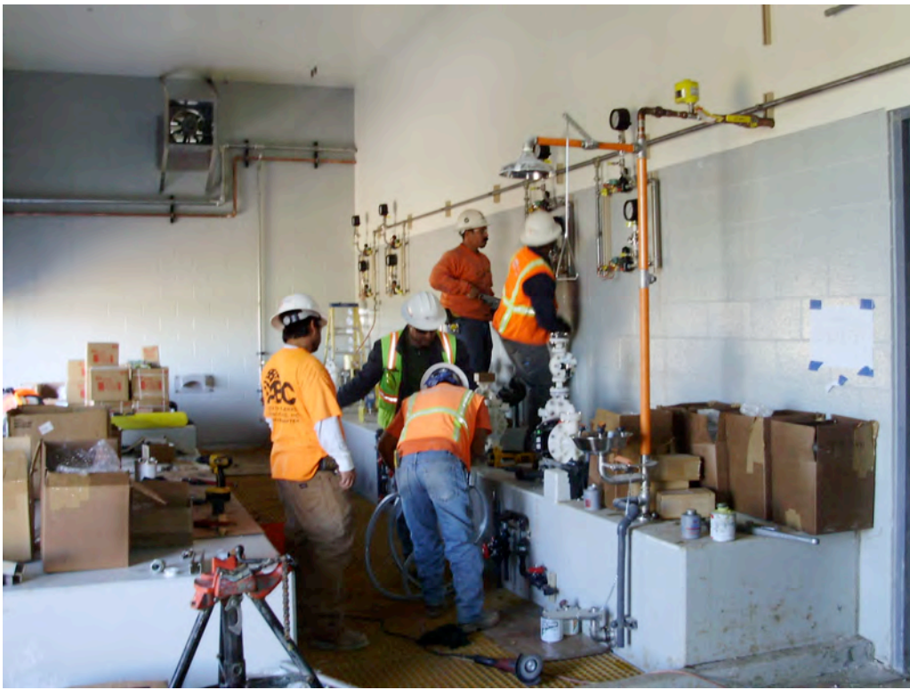
Chemical Pump and Piping Installation at Chemical/Blower Building
