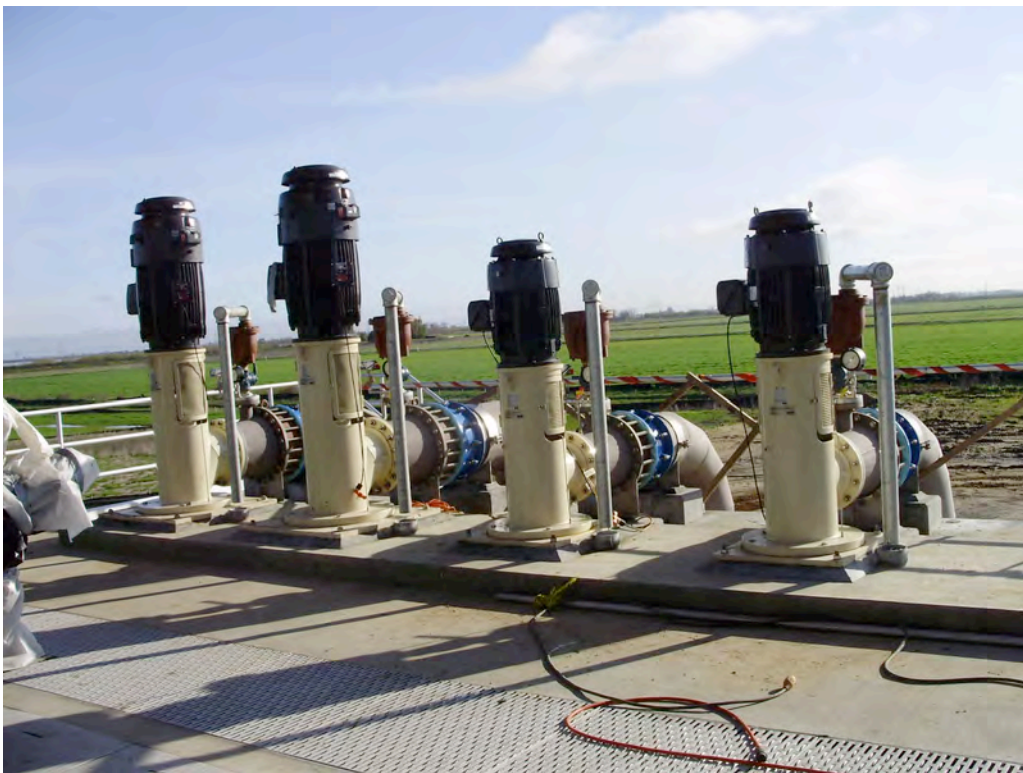
Effluent Pump/Piping Completed
