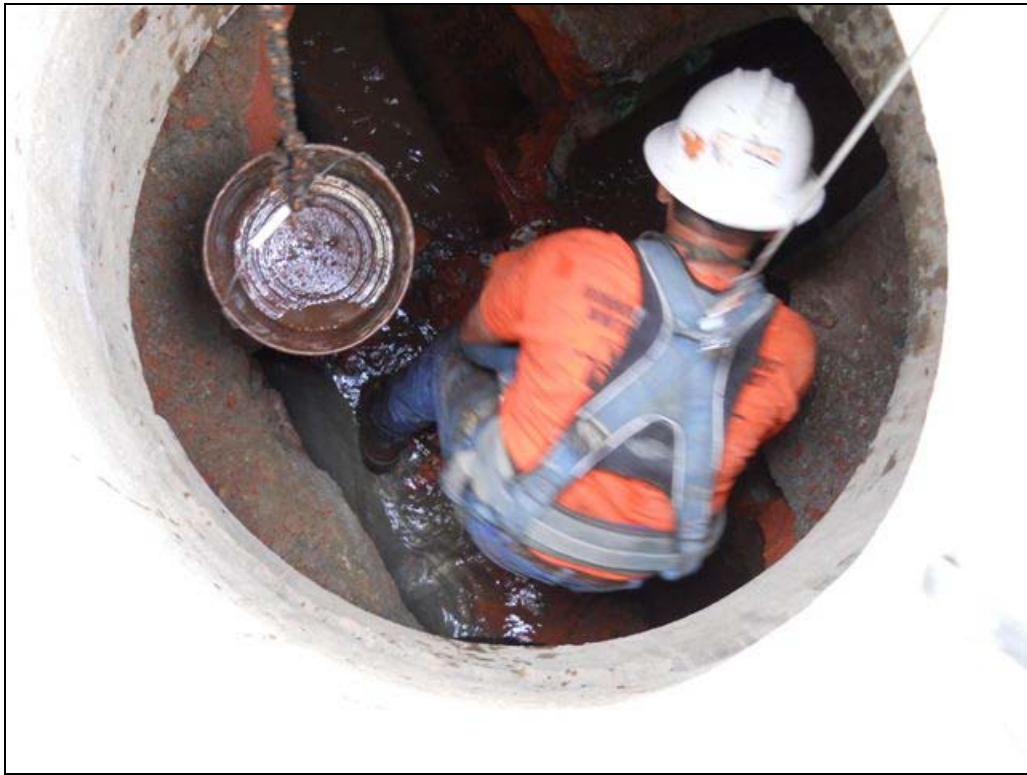
Preparing Manhole to Divert Flow to the New Treatment Facilities
