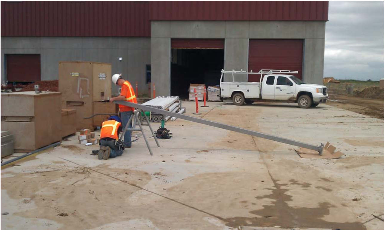
Preparation for Installation of Site Lighting
