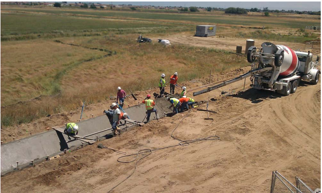
Installation of the Concrete Lined Ditch
