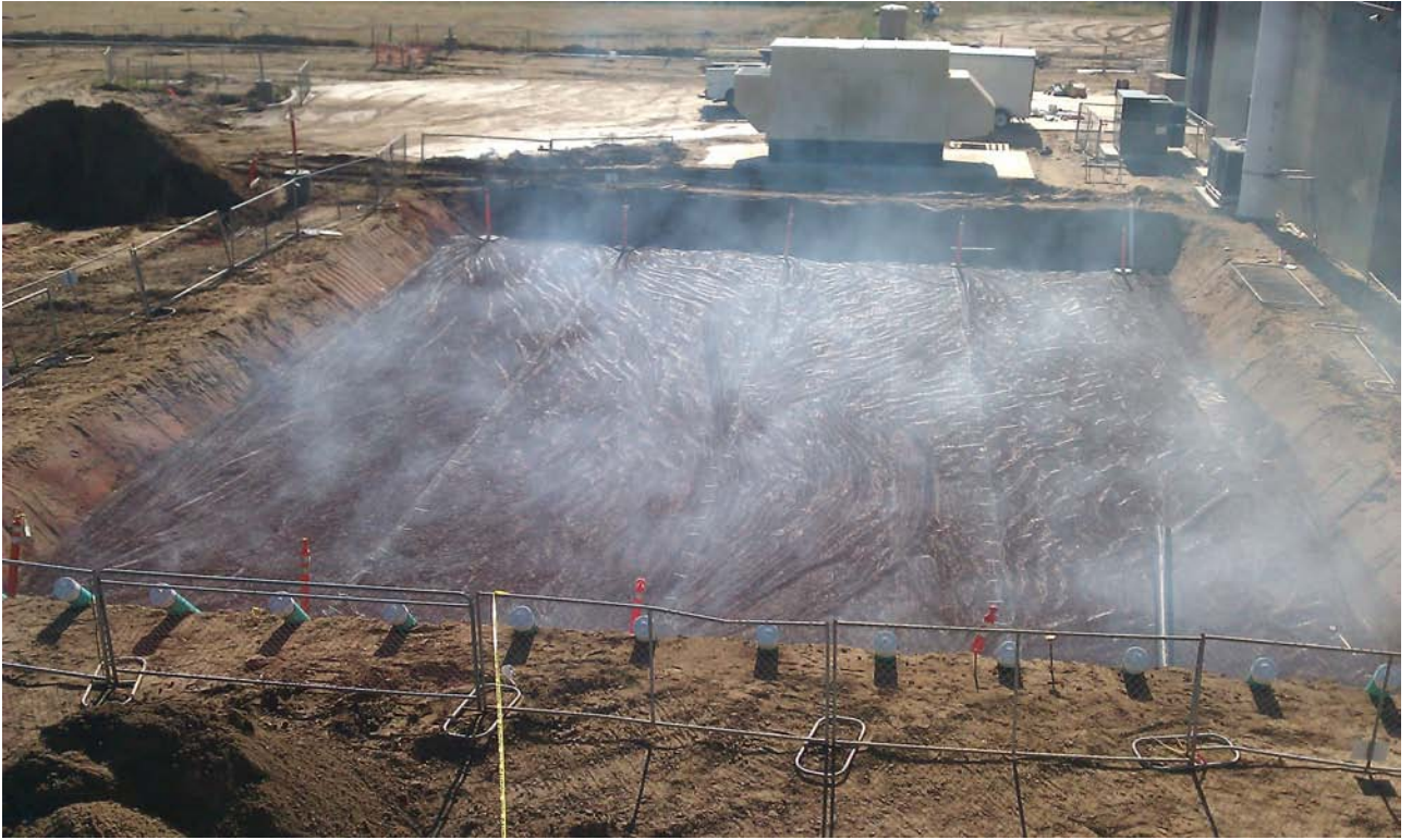
Smoke Testing the SHB Biofilter Prior to Placing the Media
