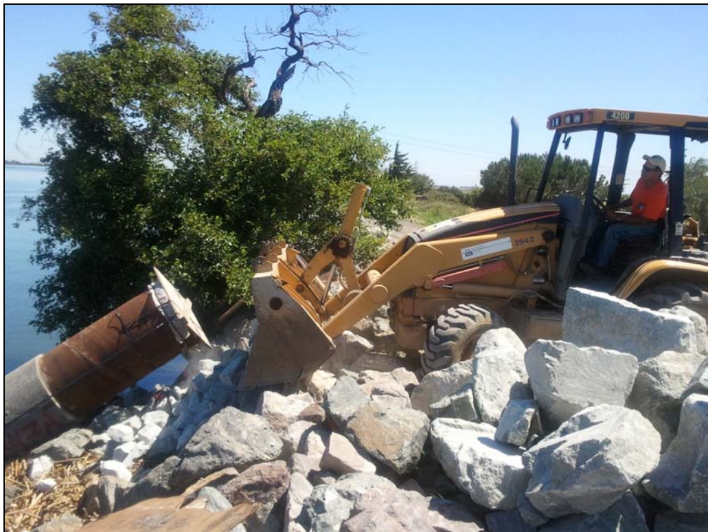
Rip Rap Placement at the Levee Slope
