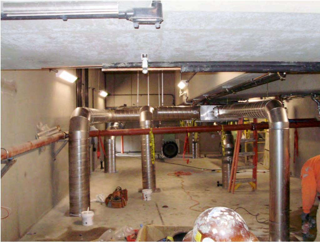
Laboratory HVAC Ductwork Installation at Headworks
