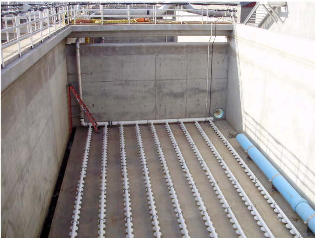
Aeration Basin Diffuser Installation
