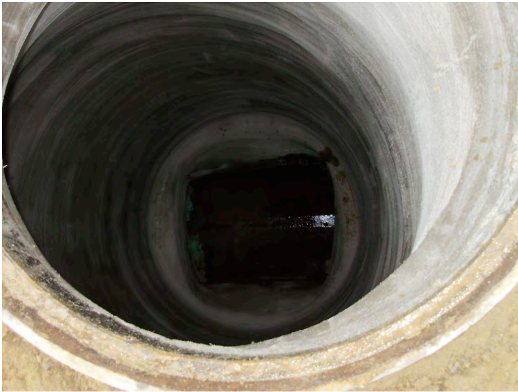
Influent Manhole Coating
