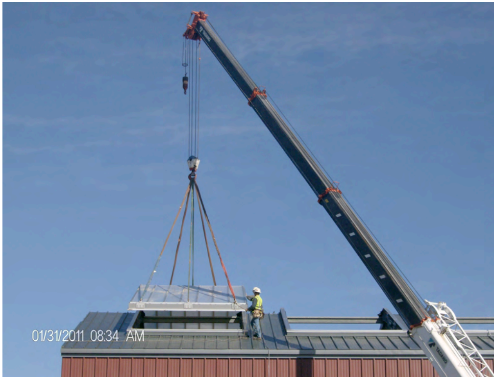
Skylight Installation at the Solids Handling Building
