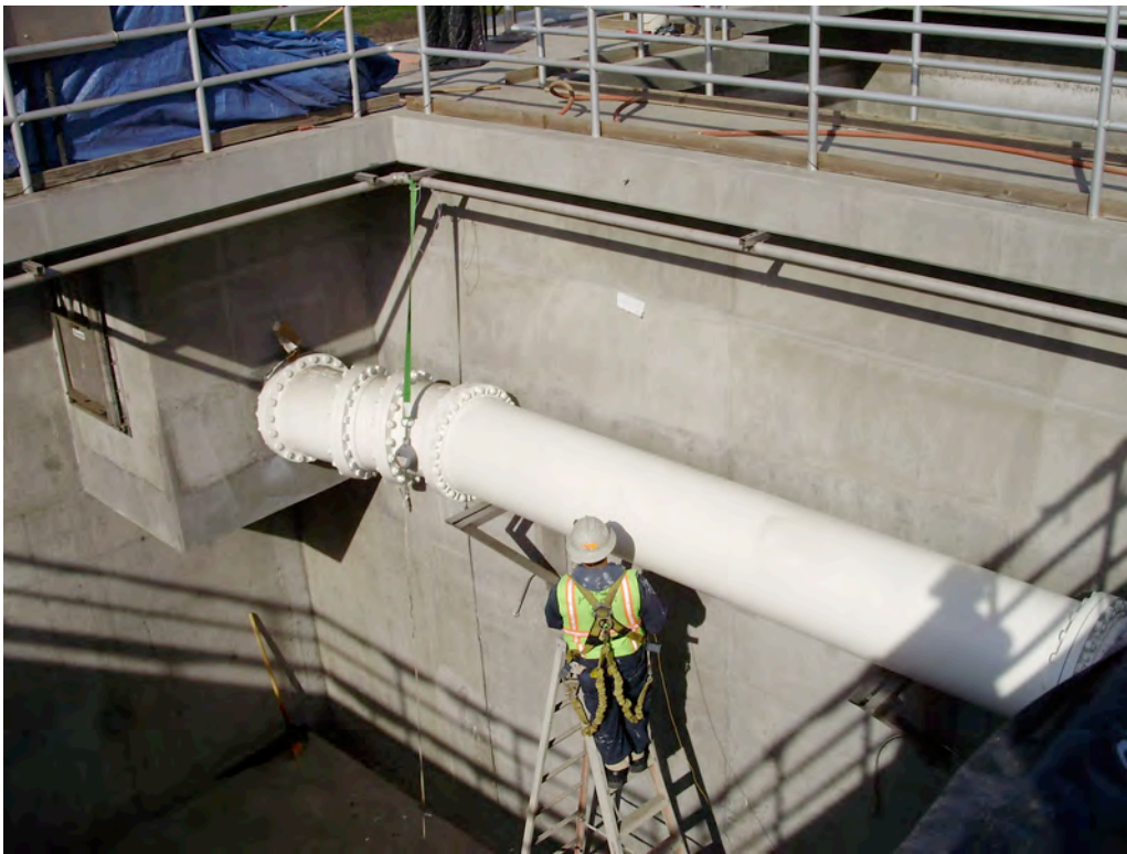
RAS Pipe Coating Inspection
