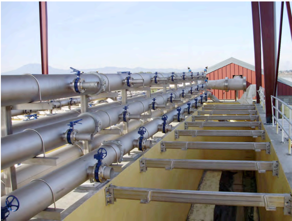
MBR Piping Installation
