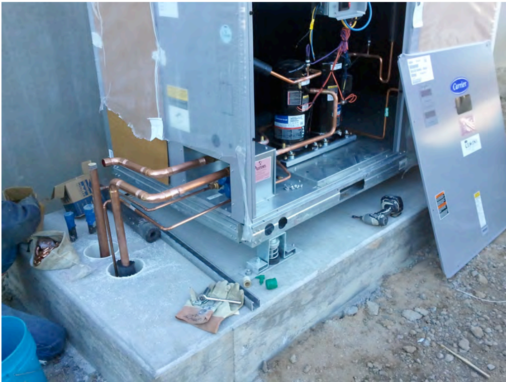
Solids Handling Building HVAC Equipment Installation
