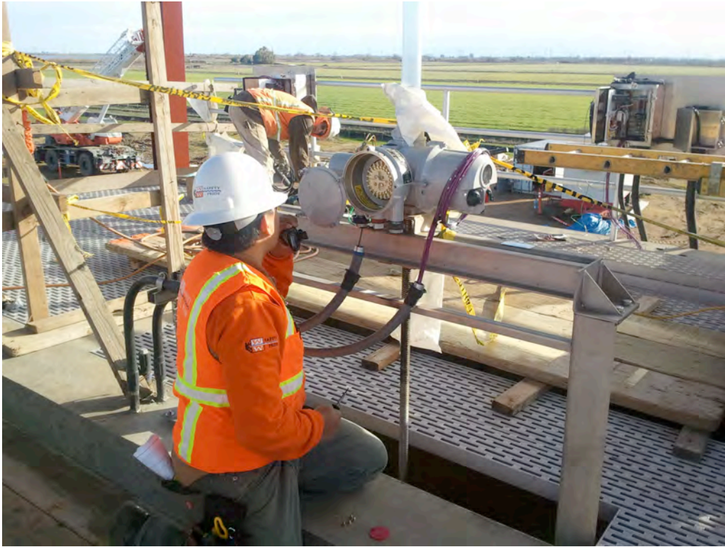
MBR Gate Actuator Wire Installation
