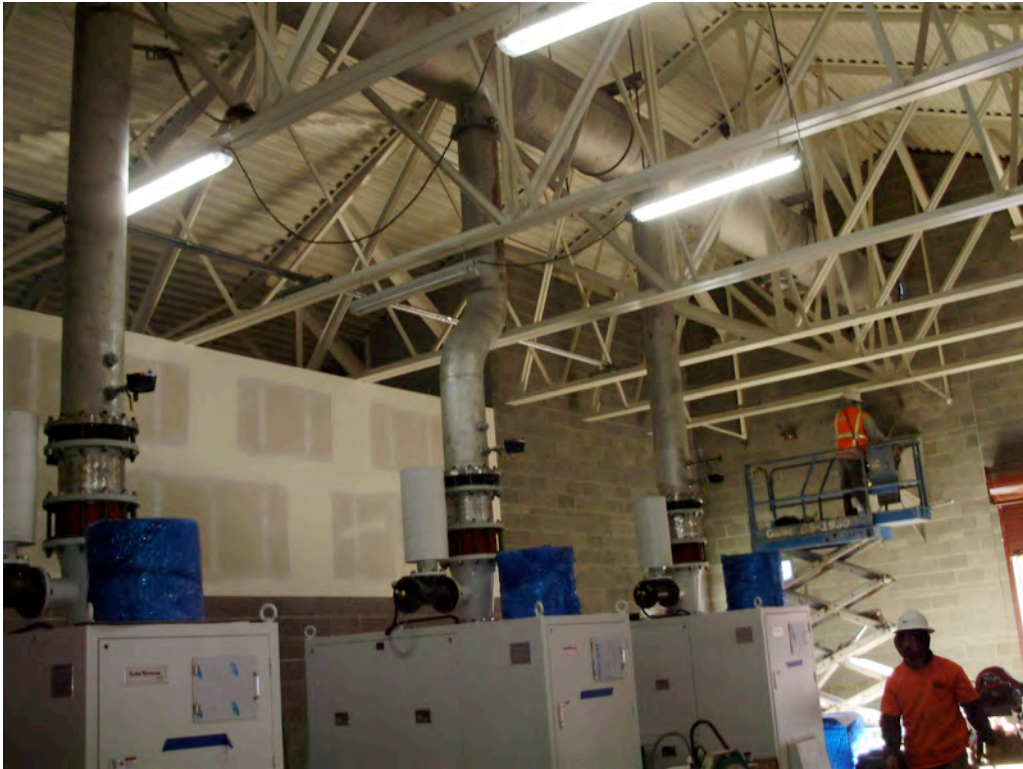
Chem/Blower Building Piping Installation
