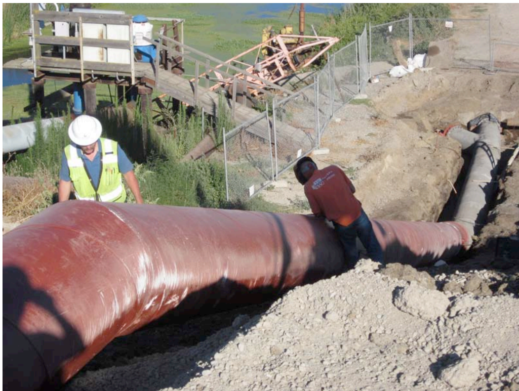
Outfall Pipe Installation
