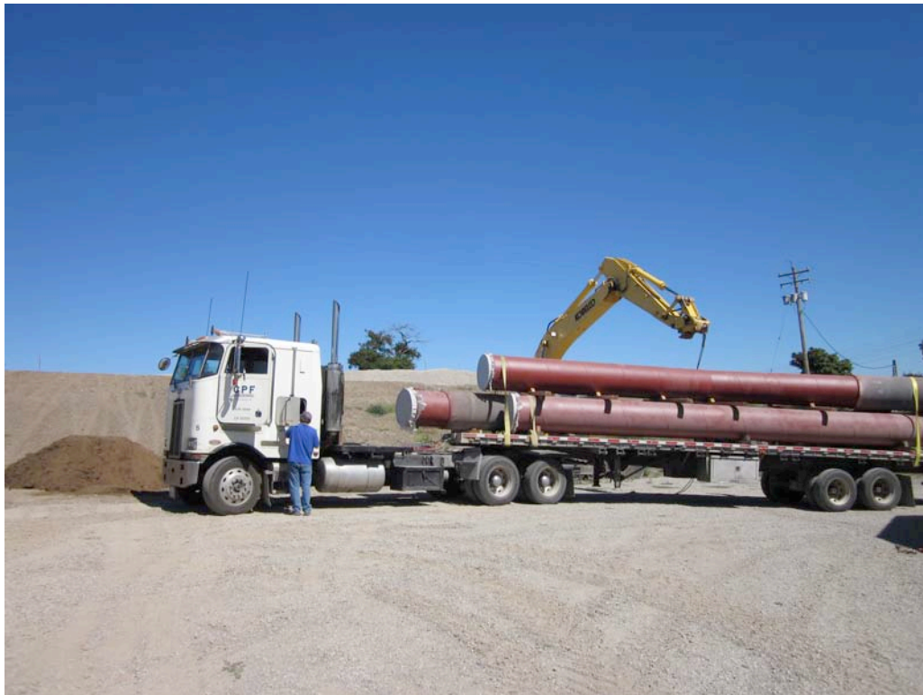
Outfall Pipe Delivery
