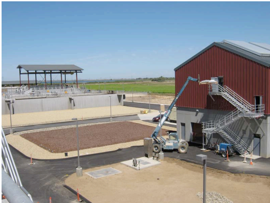
Deliver Grating to Complete Platform at Solids Handling Building
