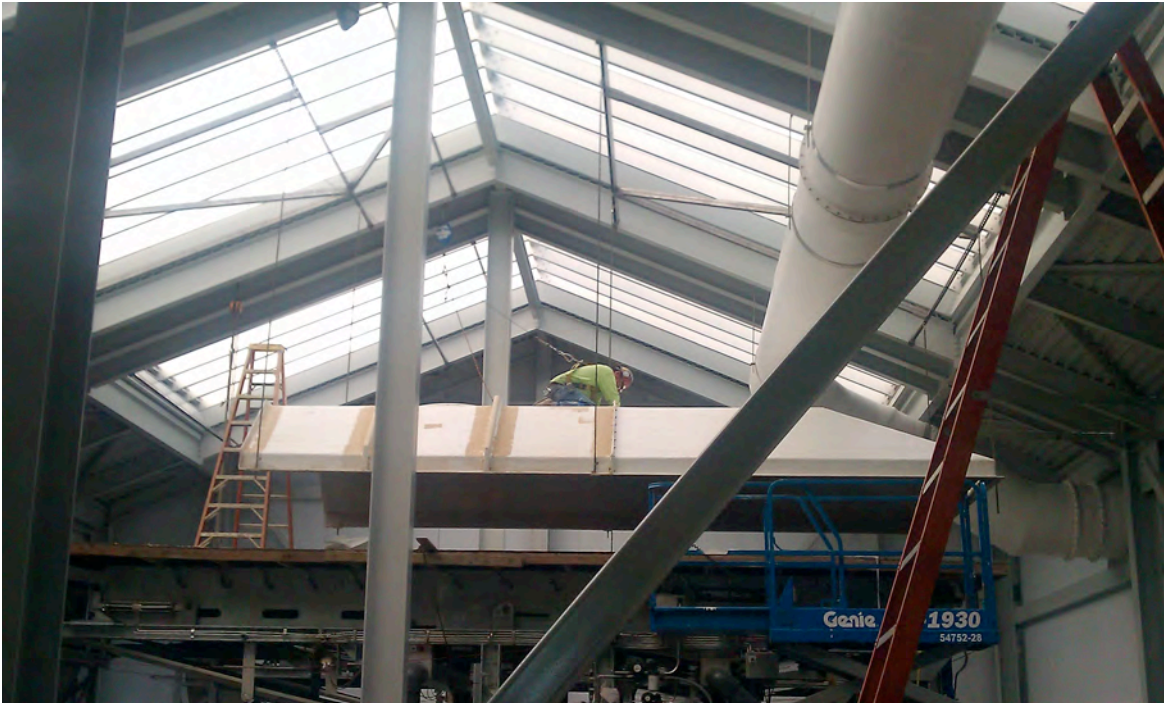
Belt Press Odor Control Hood Installation
