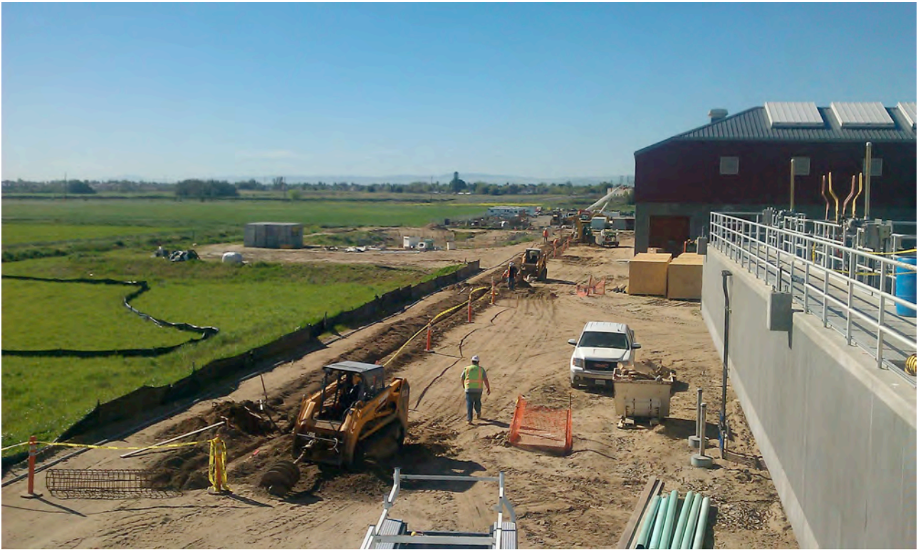
Site Lighting Ductbank and Pole Base Installation
