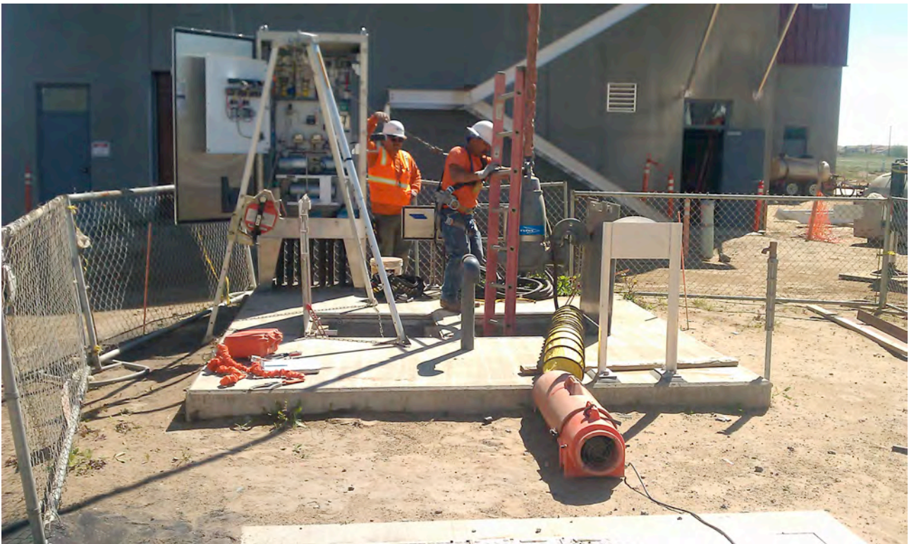
SHB Filtrate Pump Station Installation
