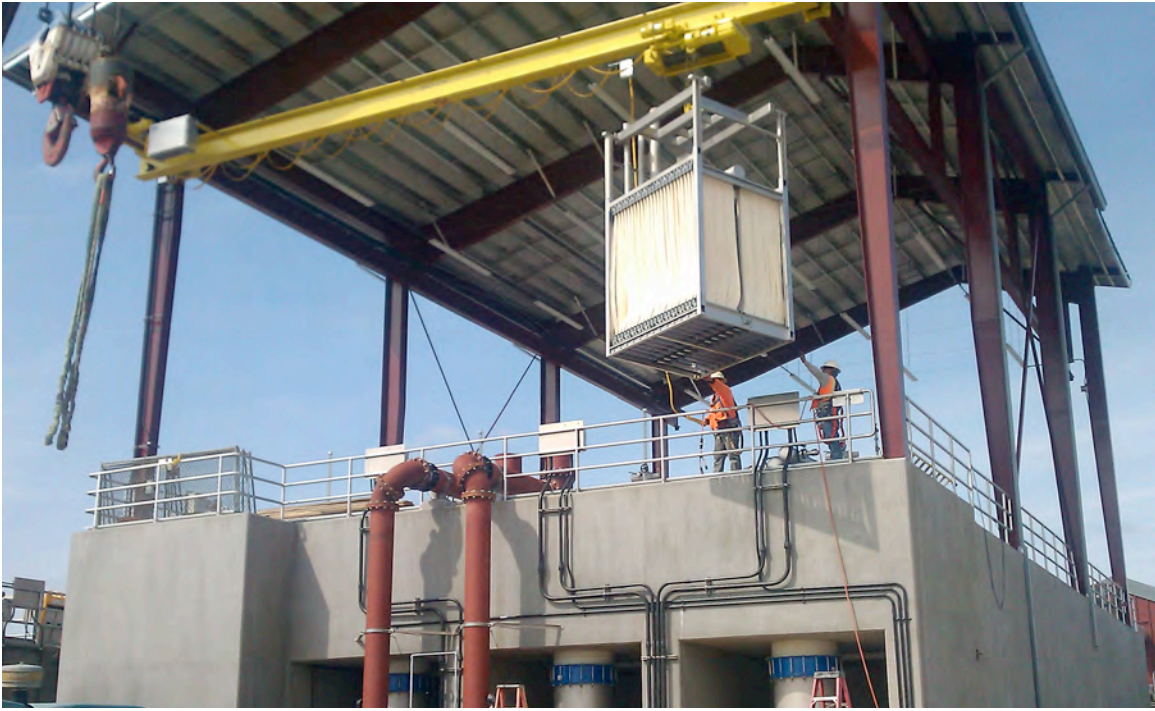
MBR Equipment Installation
