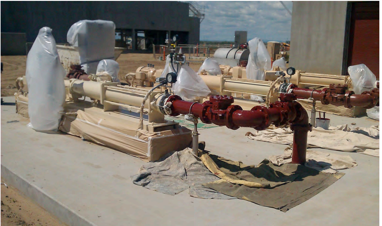
Ongoing Painting of Piping and Equipment
